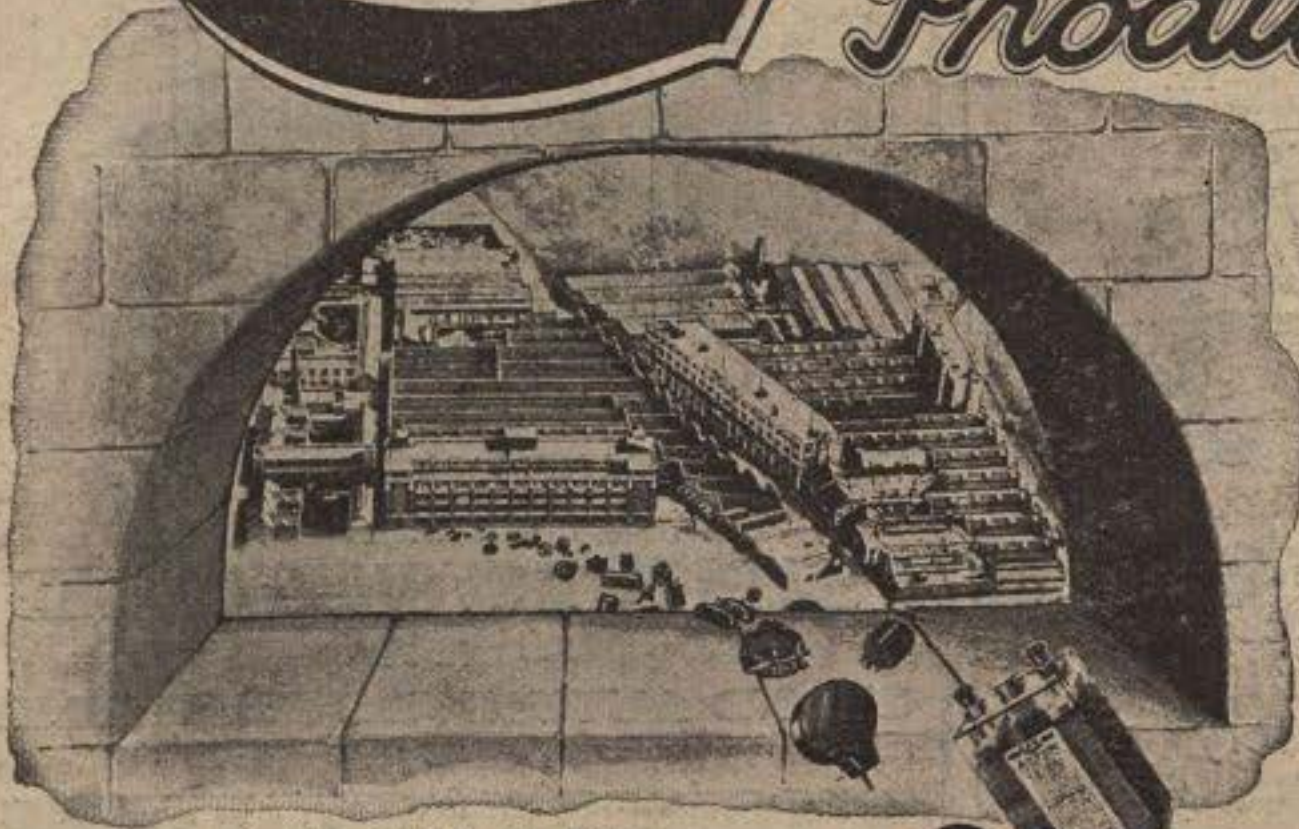
Aerial View of C.A.V. Acton Works.
